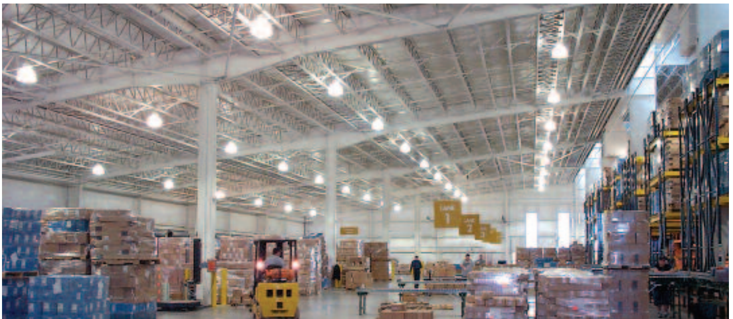
Long Bay Steel Roof Framing System
